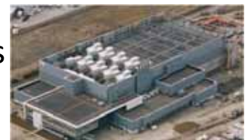
Microsoft's chiller-less data centre in Dublin, Ireland.
