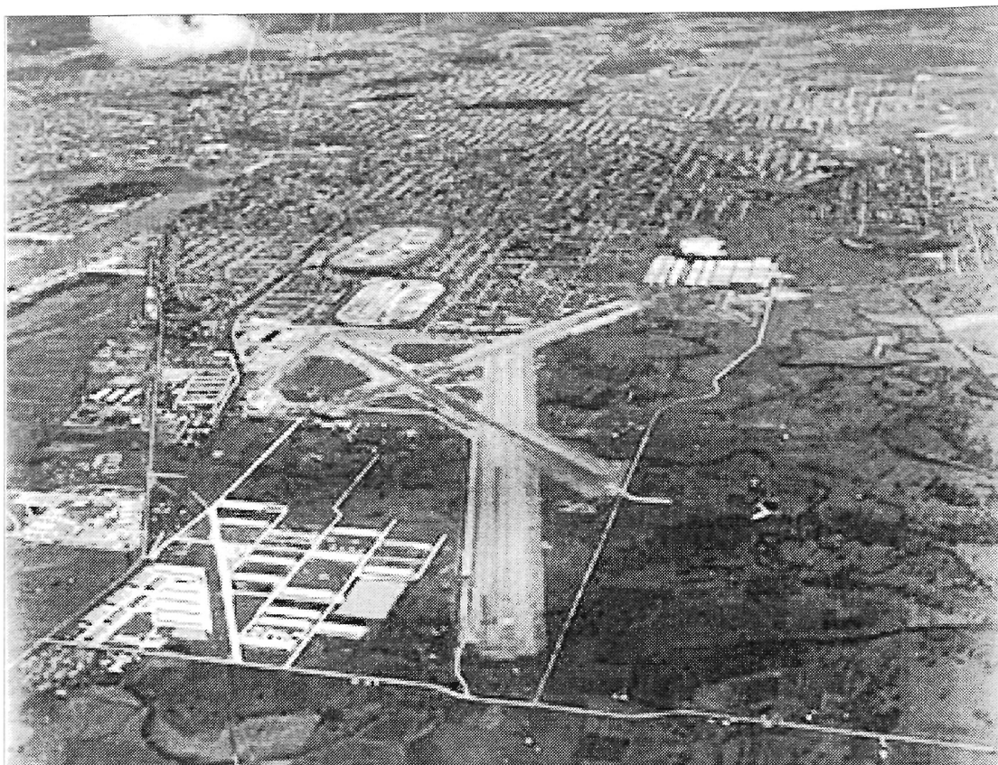
Figure 38: Aerial view of Eagle Farm Aerodrome, 9 August 1944. All three intersecting runways have been constructed.
