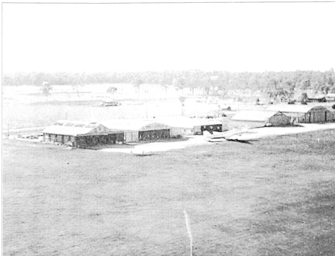
Figure 19: Aerial view of hangars and surroundings, Archerfield circa 1938. From left to right the hangars are numbers one to five. The house in the middle left distance belonged to Alex Spring. The Lorenz tower is situated between hangars no 3 and no 4. Source: Esther L'Estrange photograph album, David Molesworth Collection
