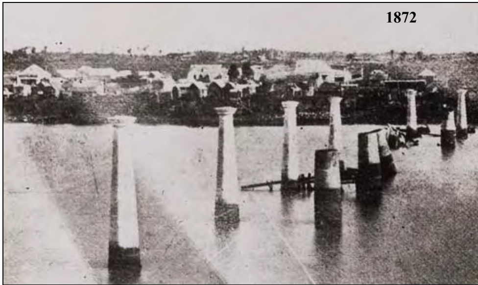
Figure 86: Old Victoria Bridge, under construction in 1872. (Source: Fryer Library, UQ)
