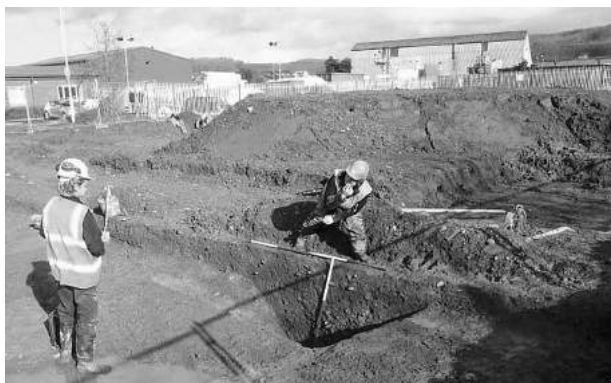
Figure 24. Ditch B looking north-east.
