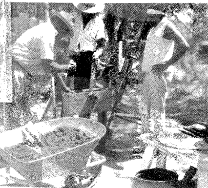
Figure 1 Manufacturing stabilised soil bricks for transitional housing in Warrabri (now Ali Curung), Central Australia, during the mid-1960s. Warrabri was one of many settlements established in the post WWII period in which to assimilate Aboriginal people. [Source: AERC Archive, University of Queensland. Photographer: B. Saini.]
