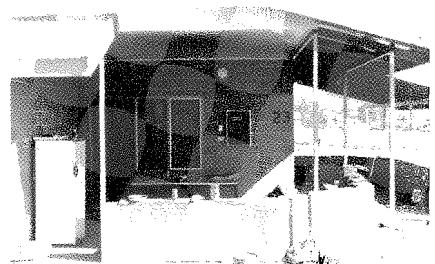
Figure 2 An example of a concrete block house provided by Tangentyere Council and designed by Dillon and Savage for Alice Springs town camps between 1984—86. The design is characterised by extensive veranda and sleep-out areas for external activities and visitor accommodation, pot belly stoves for winter heating, lockable storage cupboards, a refrigerator inside a lockable pantry, pergolas with deciduous vines, ablution rooms separable in case of effluent blockages, and security grilles. The 1987 photograph illustrates the kind of use to which an external living area was put. [Photographer: P. Memmott. Source: AERC, University of Queensland.]
