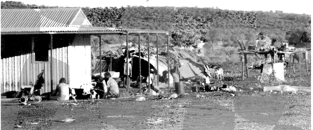
Figure 5 A Nomad house positioned alongside a Warlpiri jilimi in May 1987. [Photographer: P. Memmott. Source: AERC, University of Queensland.]
