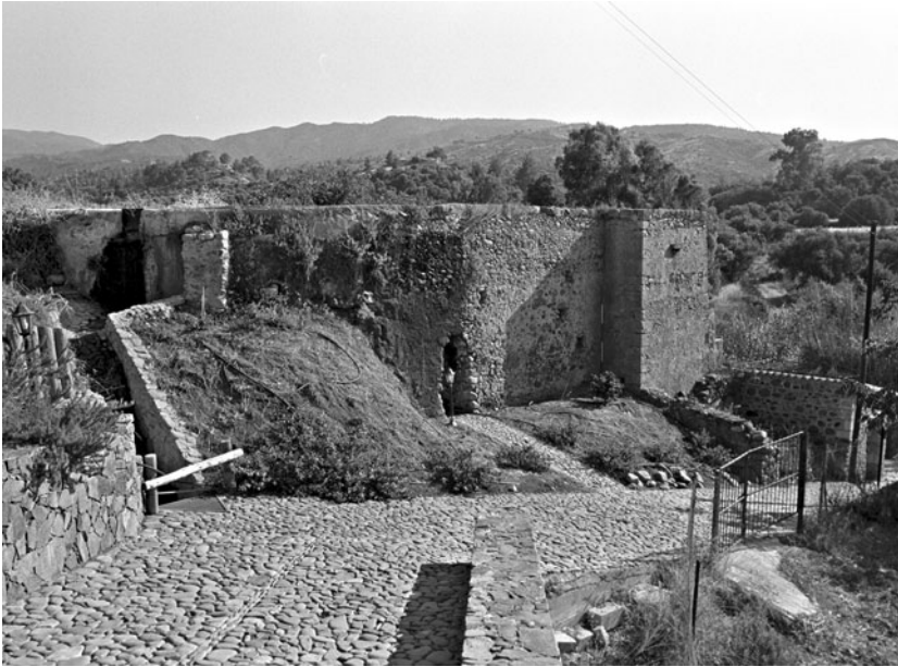
Figure 3 Molos watermill (1690). The water passes along the aqueduct from the left to the penstock on the right. The cross and inscription (figure 6) lie directly under the projecting block in the side of the penstock (Chris Parks).
