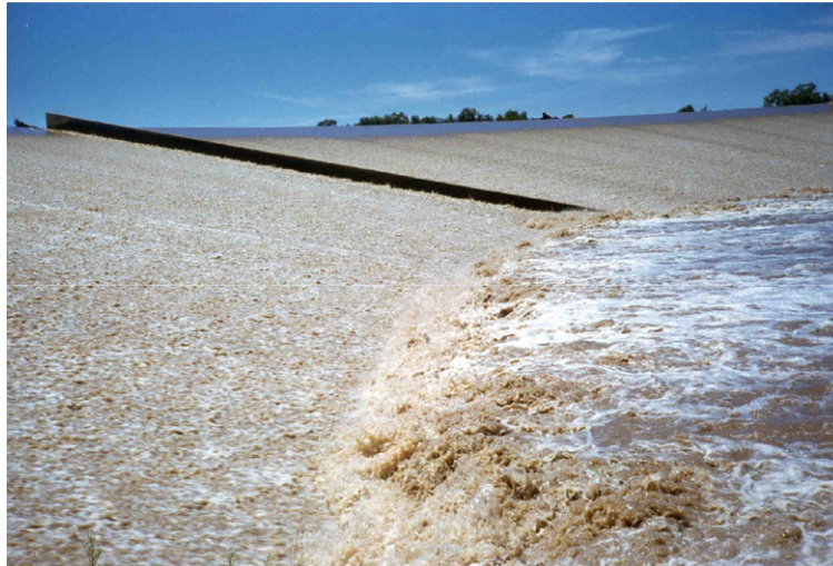
Fig. 18. Hydraulic jump at the spillway toe of Chinchilla minimum energy loss weir on 8 Nov. 1997.
