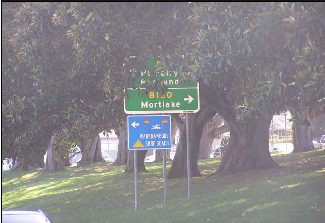
Figure 16: Regular pruning may be required to ensure sign visibility
