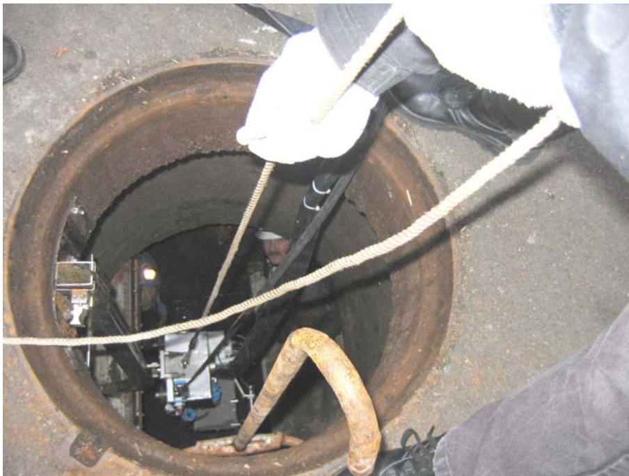
Figure 4 - Installation of the two-dimensional sampler through a manhole
