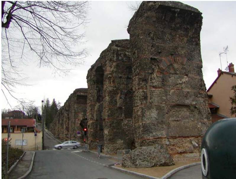
(D) Gier aqueduct (Lyon, Fra.) - Inverted siphon structure of Beaunant downstream of the arcades du Plat de l'Air - The masonry structure supported 11 (or 12) lead pipes ( \varnothing_{\text{ext}} = 230 \text{ mm} , \varnothing_{\text{int}} \approx 162 \text{ mm} ), the maximum drop in elevation was 122 m and the total length of the siphon was 2660 m - Looking upstream at the 270 m long bridge supporting the pipes
