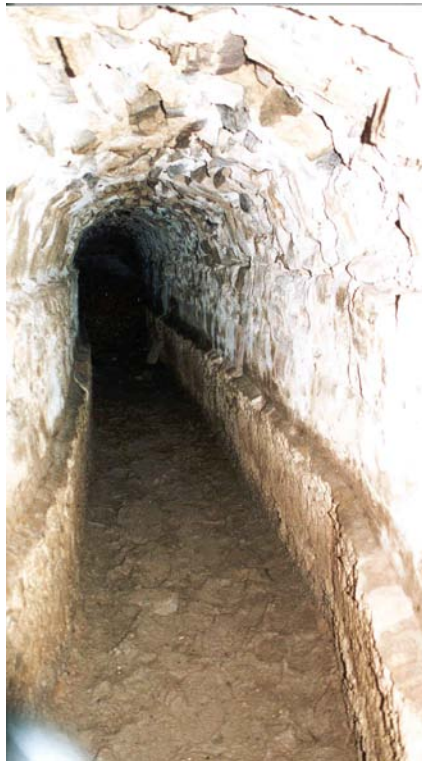
(B, Left) Brévenne aqueduct (Lyon, Fra.) at Bitermay - Inside view of the subterranean conduit - The internal height of the conduit was about 1.7 m
