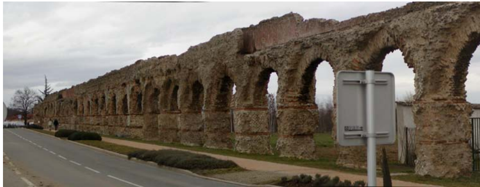
(A) Gier aqueduct (Lyon, Fra.) - Elevated channel and arcades du Plat de l'Air at Chaponost - The arcades are 55 m long and up to 15 m high and include 92 arches
