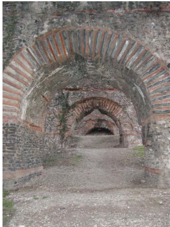
(B, Left) Brévenne aqueduct (Lyon, Fra.) at Bitermay - Inside view of the subterranean conduit - The internal height of the conduit was about 1.7 m
