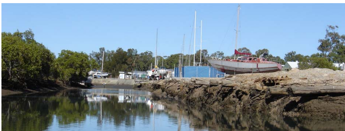
Figure 1.1 – Boat repair yard located in Erapah Creek, Australia. Photograph taken mid ebb tide (09:41) on 7/06/06 during field study E7 (5-7/06/06).
