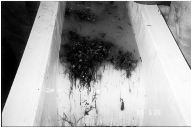
Figure 5 – Weed Flow over Weir Crest
