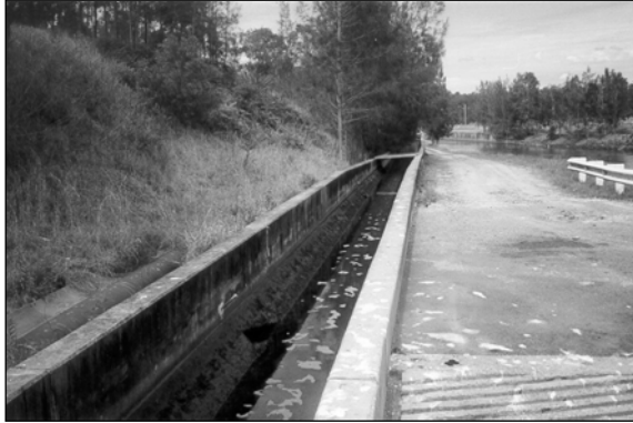
Figure 2 - Section of Trapezoidal Channel
