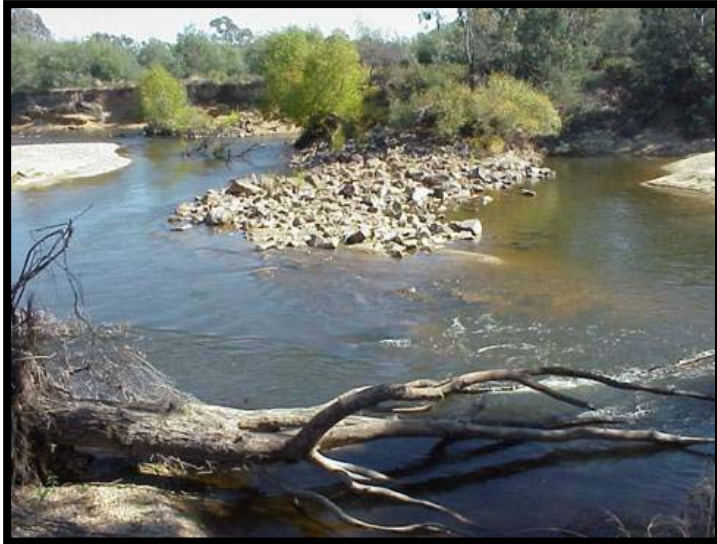
Figure 5 – A large rock chute outflanked when river banks eroded
