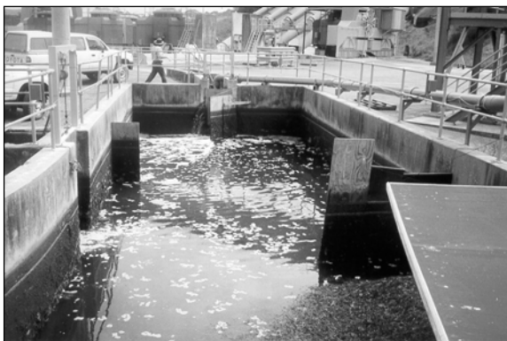
Figure 1 – Weed-Settling Pond (Pre-modification)
