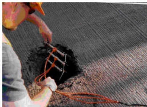
Figure 5 Cluster of 3 gauges being installed in highway pavement.
