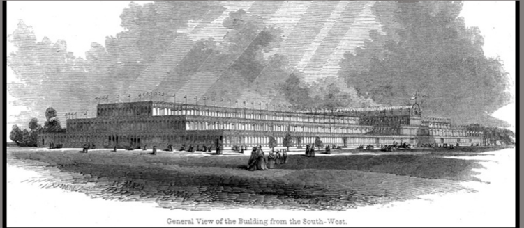
General View of the Building from the South-West.
