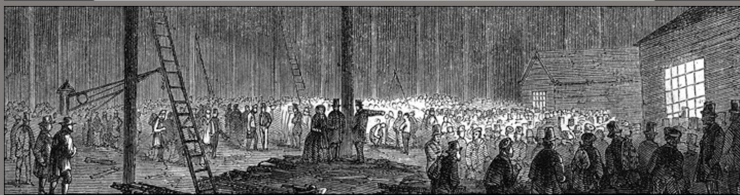
Workmen waiting to be paid. Over 2000 were employed on the site at some periods.
