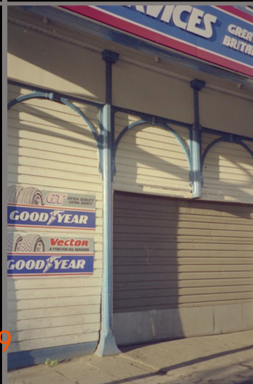
Iron column - every third 8' bay
