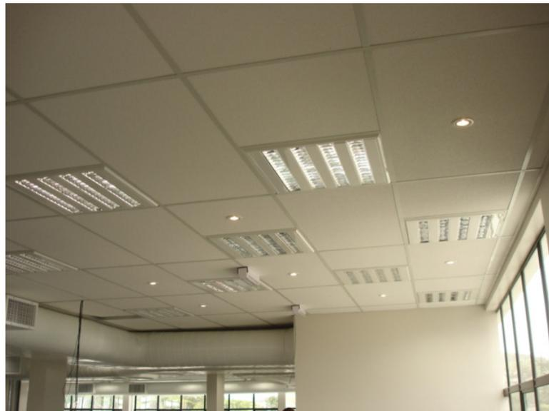
**FIGURA 14 – FORRO TIPO FIBRA MINERAL**
