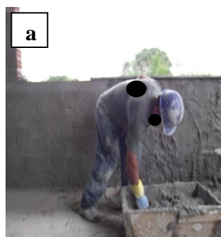
a Pegar a argamassa na padiola
