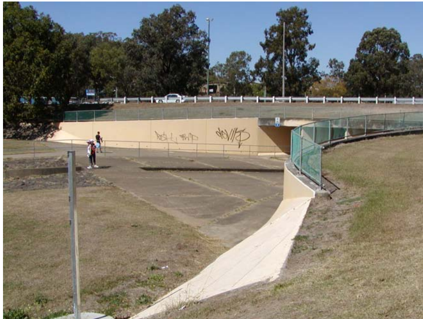
Fig. 5 - Operation of the Ridge Street Minimum Energy Loss culvert on Norman Creek
