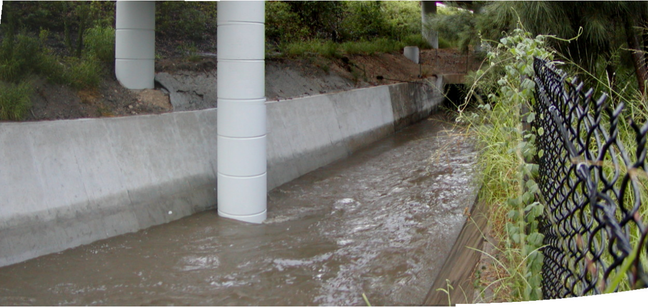
Fig. 6 - Inlet of the Minimum Energy Loss culvert at Marshall Road, Brisbane at the end of a storm on 31 Dec. 2001 - Looking downstream at the inlet flow with one of the concrete piles
