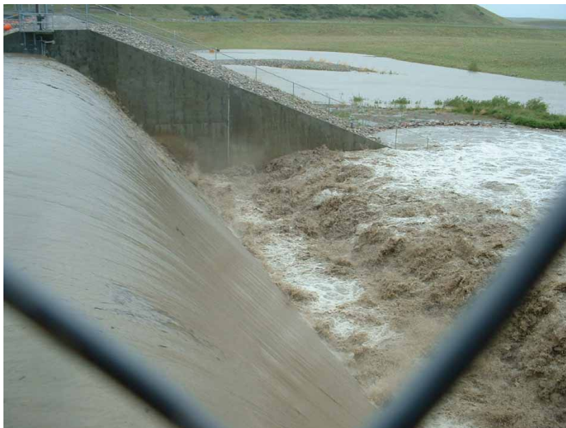
Figure 1. Photograph of a hydraulic jump energy dissipator in operation (Courtesy of John REMI) - Pine Coulee dam spillway during floods in South Alberta, Canada in June 2005 - Flood flow from left to right.
