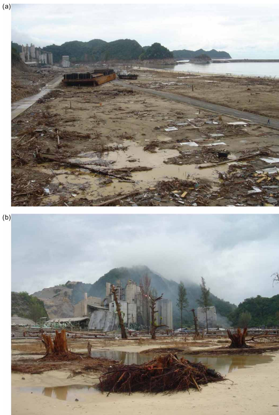
Figure 3. Photographs of a damaged cement plant in the Lhonga Area (South-west of Banda Aceh) after the 26 December 2004 tsunami disaster (Photographs Dr V. GUSIAKOV, Novosibirsk Tsunami Laboratory) (A) Looking South from a hill top at a tug boat and large barge moved inland by the tsunami waves, with the cement plant in the background left and a sunken ship in the harbour (background right) (B) Damaged cement plant.
