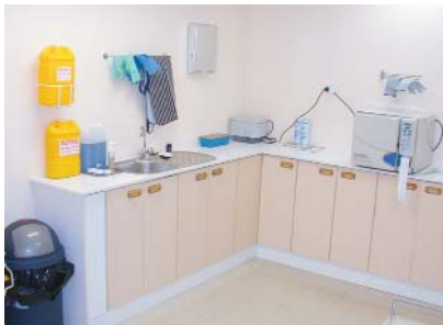
Figure 10. When planning a sterilizing room, consideration must be given to adequate lighting for the high detail tasks such as inspecting instruments after cleaning. Normal ceiling lighting, which is placed centrally, gives shadows for work undertaken on benchtops. This layout with no natural lighting would benefit greatly from wall mounted lights with pelmets above the sink area.
