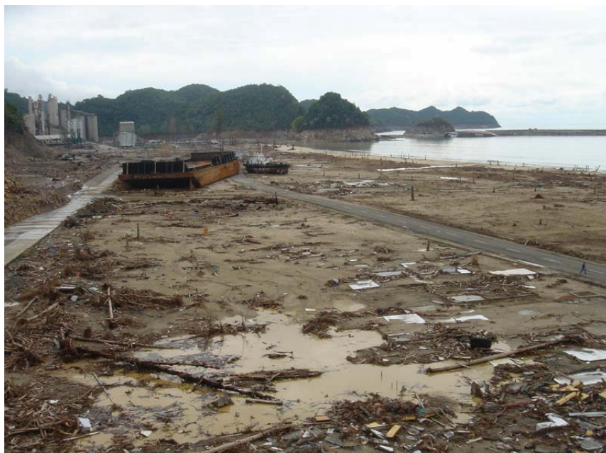
(B) Damaged cement plant in Western Aceh after the 26 December 2004 tsunami disaster (Photograph of Dr V. Gusiakov, Novosibirsk Tsunami Laboratory)
