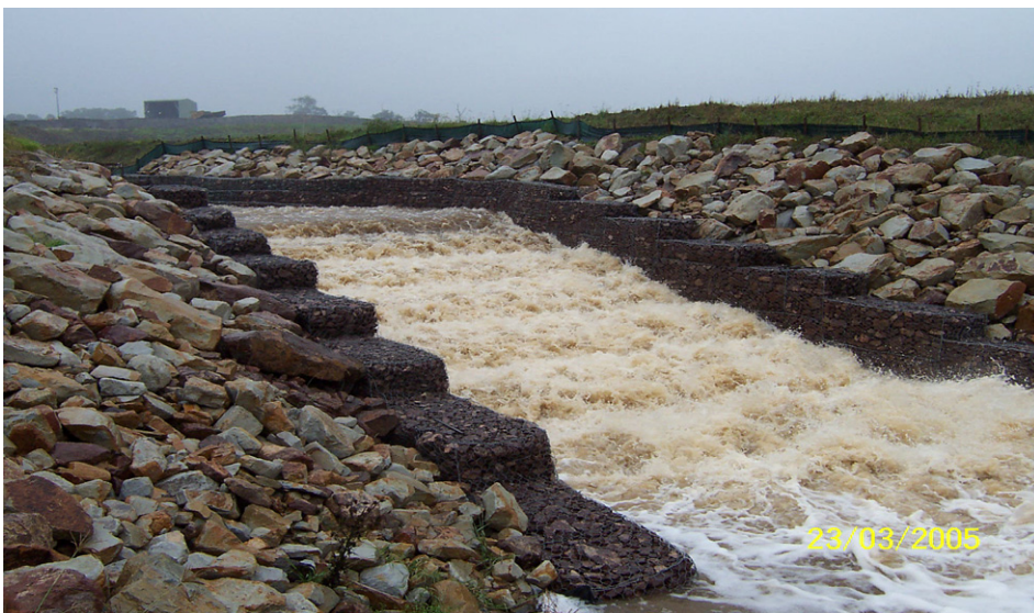
Fig. 1. Photograph of rough stepped chute flow at Duralie coal mine stepped spillway NSW, Australia on 23 March 2005 (Courtesy of Tony MARSZALEK, Gilbert & Associates Pty LTD, Brisbane) – Slope: 1V:5H, h = 0.5 m, gabion construction.
