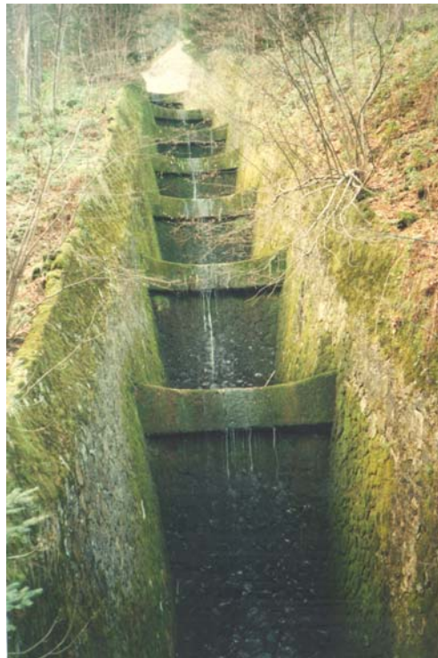
(b) View from downstream of the masonry stepped spillway located on the left bank.
