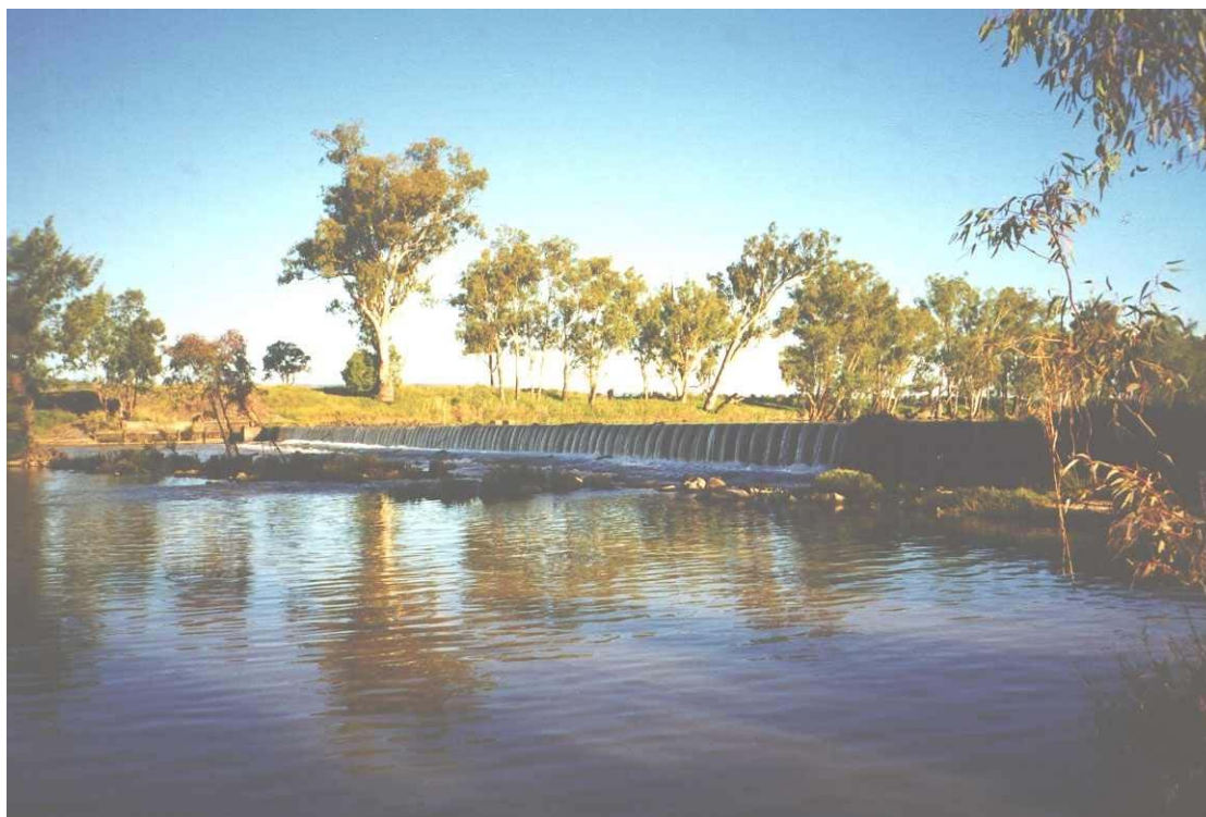
(C) View from the present weir from the left bank : note the ruins of the first weir in the foreground, downstream of the sheet-pile cascade (Photograph taken in February 1998)
