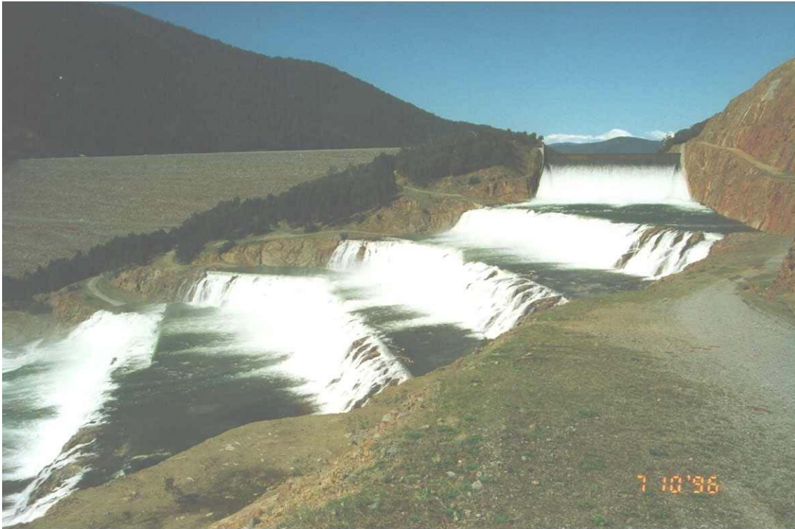
Fig. 6 - Dartmouth dam spillway during the 1996 overflow ( Q_w \sim 225 \text{ m}^3/\text{s} ) (Courtesy of Mr JEFFERY, Goulburn-Murray Water) (B) Details of the cascading flow from the left bank, showing the concrete-lined chute and the first steps
