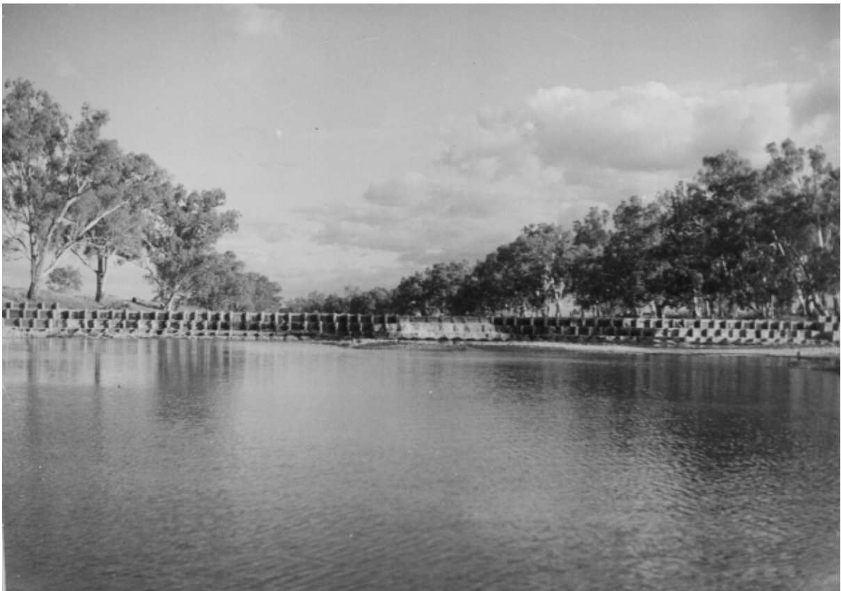
(A) First Bonshaw weir around 1953, view from downstream (Courtesy of the Department of Natural Resources)
