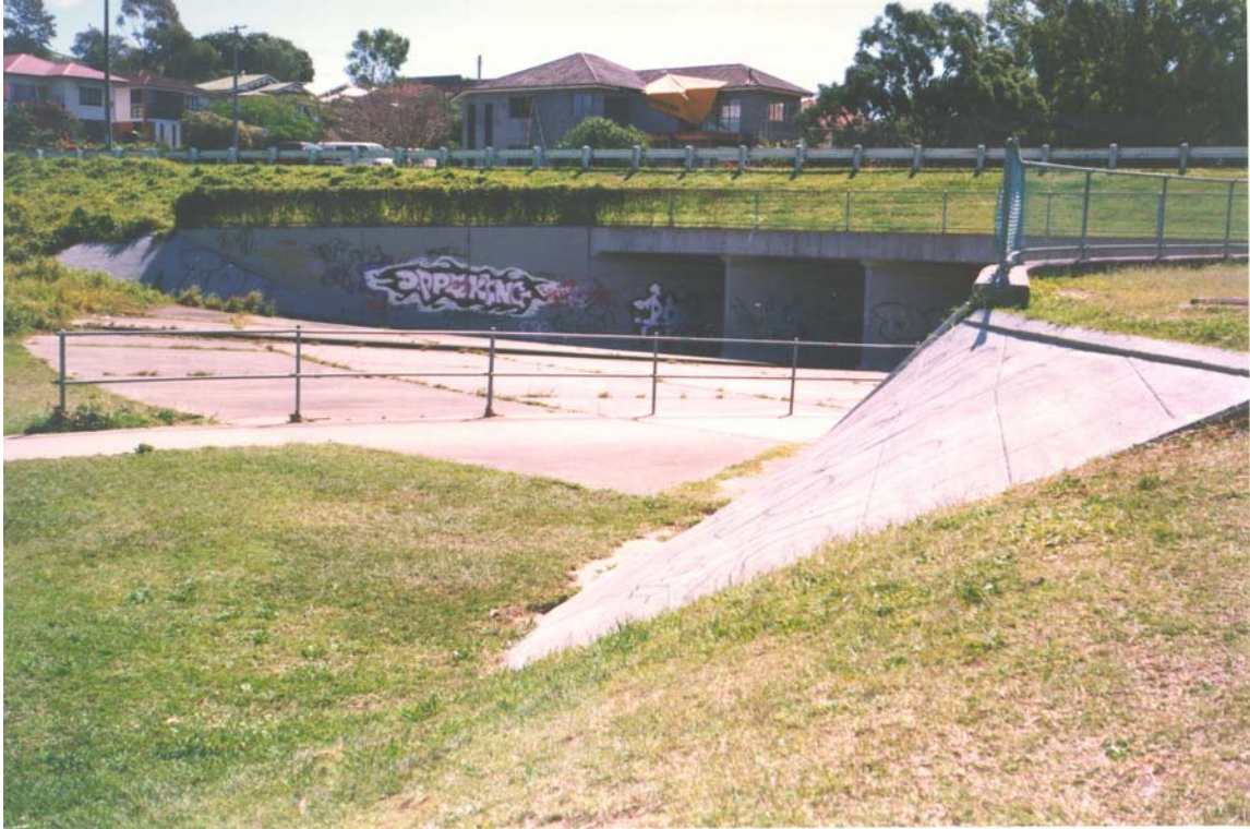
Fig. 4 - Photographs of a prototype MEL culvert below Ridge Street, Brisbane QLD, Australia - Design discharge : 220 m 3 /s; Barrel : 7 cells (2-m wide each)
