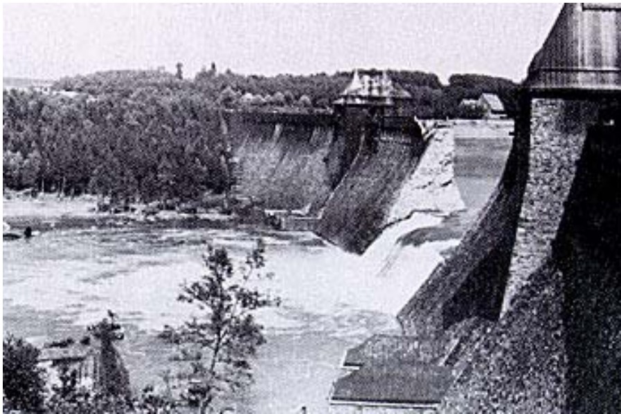
Fig. 3-1 - Photograph of the Möhne dam break (17 May 1943) - View from the left bank
