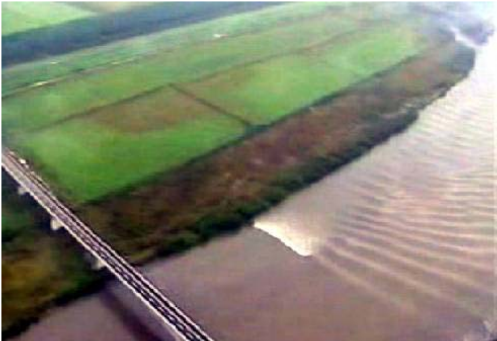
Figure 6-6 -Tsunami-induced bore during the 2003 Tokachi-oki tsunami in Japan (Courtesy of Professor SHUTO, with assistance of Prof. Kenji SATAKE) - Bore propagation from top right to bottom left - The bore propagates upstream toward the bridge
