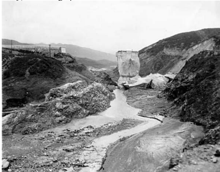
Fig. 6-1 - Example of instantaneous dam break: the St Francis dam, USA (Courtesy of Santa Clarita Valley Historical Society) - Looking upstream at the dam wall ruins
