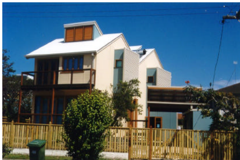
Figure 1: Prosser House, prototype environmental home
