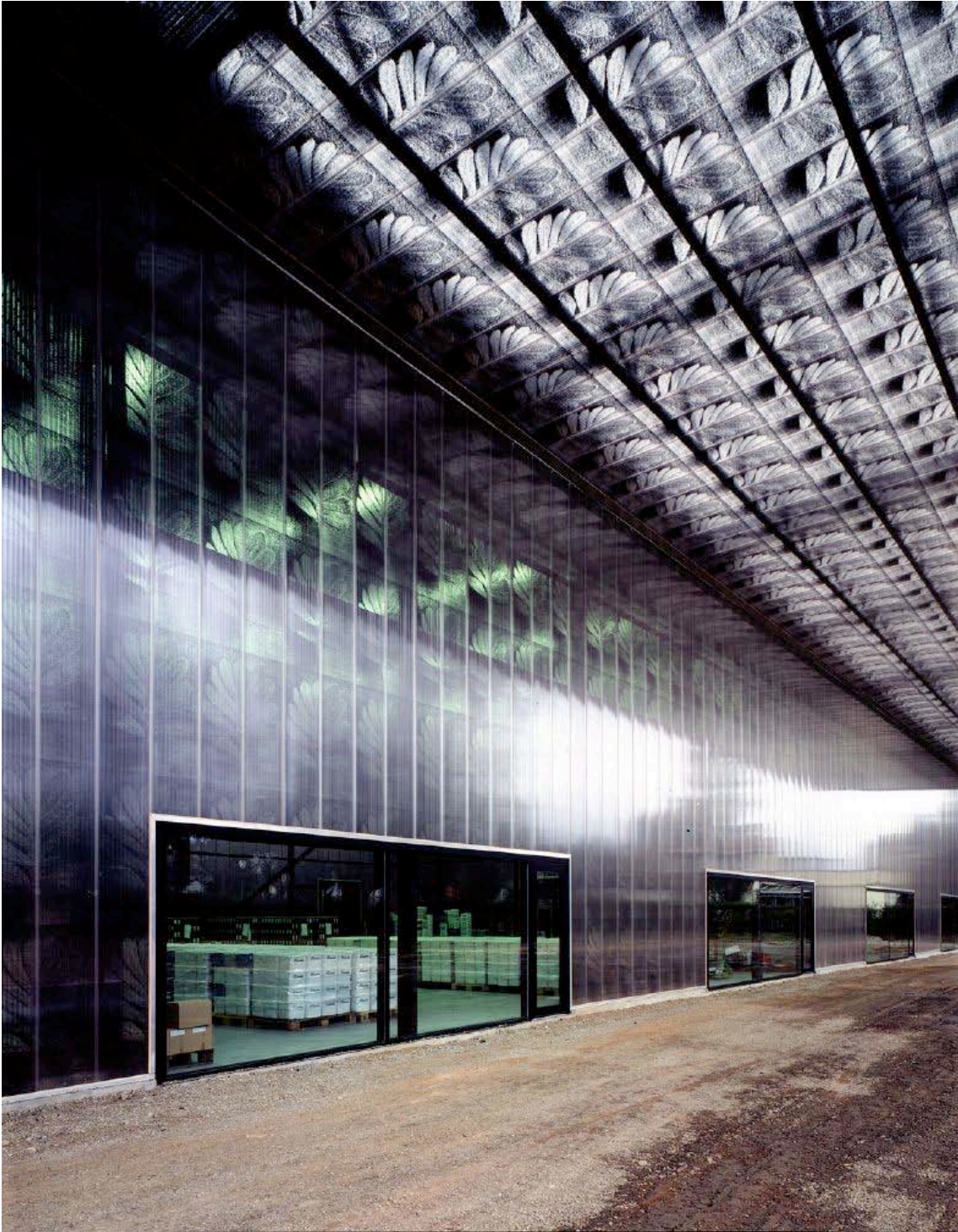
Figure 1. Herzog and de Meuron, architects, Ricola Europe SA, Production and Storage Building, Mulhouse, France, 1994. Photograph by Margherita Spiluttini. Copyright © 1994 Margherita Spiluttini. All rights reserved.
