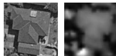
Figure 4: One of the buildings in the test dataset. Left: Digital orthophoto (resolution: 15 cm). Right: DSM.
