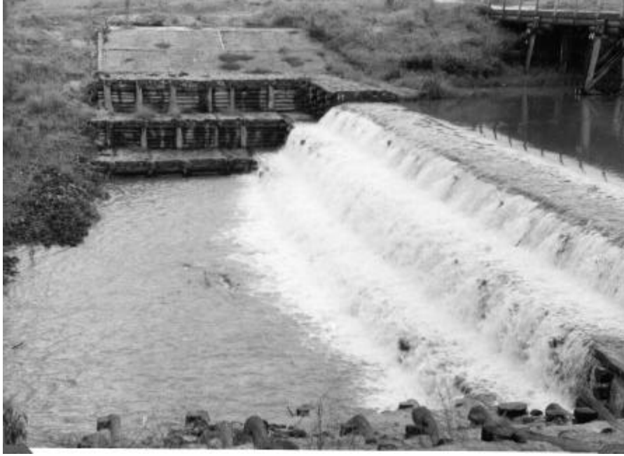
Fig. 3-1 - In-stream re-aeration cascade : Emerald Creek weir (Australia, 1947) in 1951 (Courtesy of Qld Dept. Natural Resources, Dam Safety) - Weir : H = 5.2 m, L = 79.5 m, 3 steps, timber crib held with timber piles
