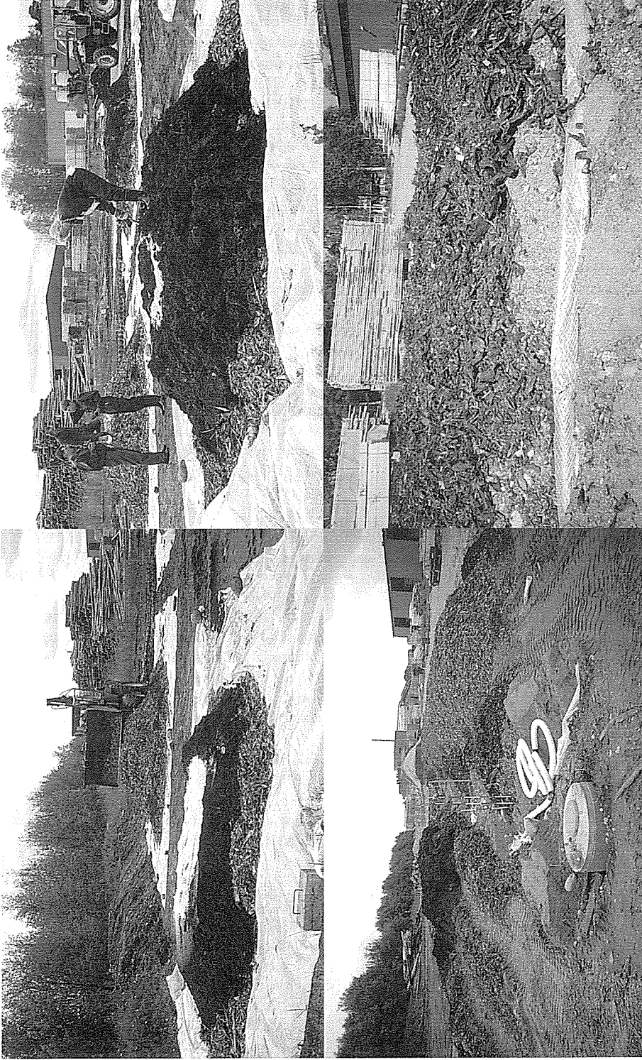
Fig. 2a. Build-up of composting. Top: Pilot piles were made from soil, bark or straw compost, lime, and nutrients in a sandwich-type (photos: K. Jørgensen). Bottom: Full-scale piles were constructed on on plastic beds which had an inclination towards separate underdrainage, and which were each covered with a 0.5 m insulation layer of bark (photos: R. Hansen).
