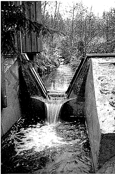
Fig. 7. Manual and automatic sampling at the measuring weirs of the catchments Rudbäck and Huhtisuonoja.
