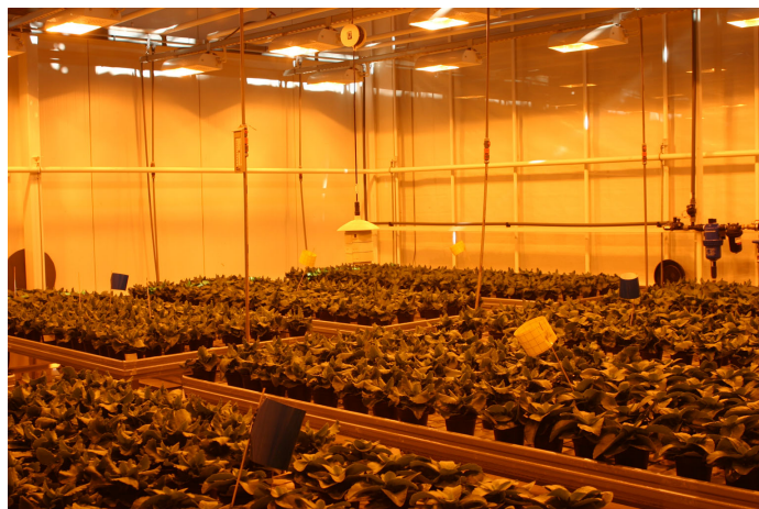
Figure 4.2: High pressure sodium lamps in a greenhouse in which sunlight is blocked to simulate natural Finnish winter light conditions. Photograph: © Valoya Oy.
