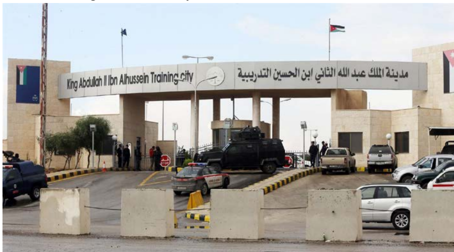
10 11 Entrance to the International Police Training Center in Amman, Jordan
