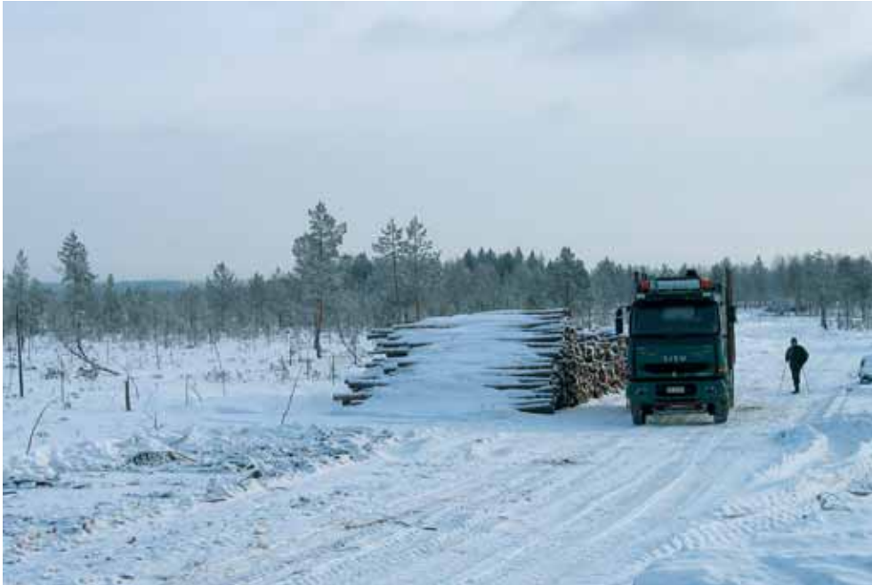
Figure 2. The restoration of originally open mire usually involves felling most of the trees in a given area. Tree removal from mires is easier during the winter, when it is possible to create a frozen winter road over the mire for the trees to be trucked out. Photo Jere Ekosaari, 9.2.2004, Haapasuo nature reserve, Central Finland.
