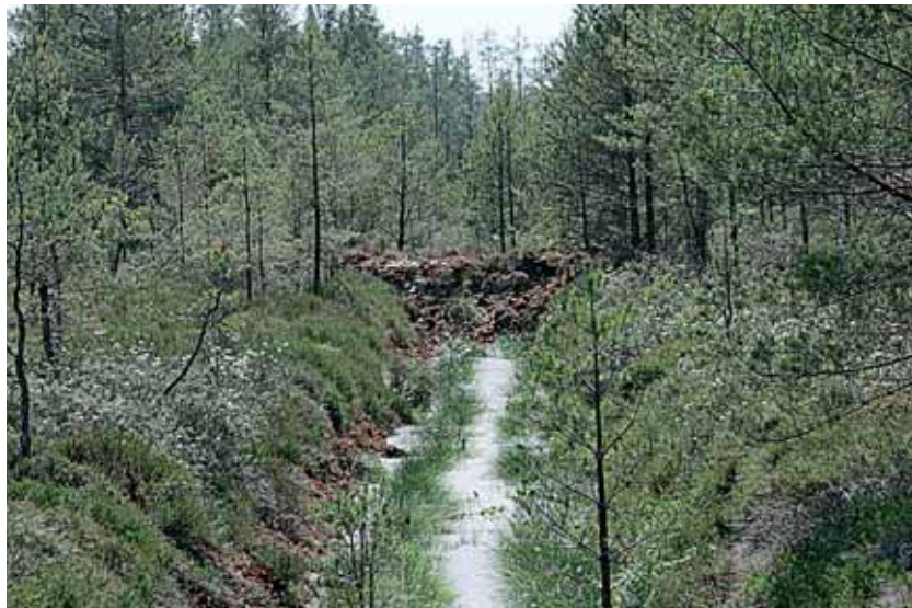
Figure 7. A dam in a drainage ditch in Vasenieki Mire (Photo M. Pakalne).
