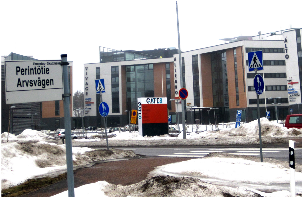
Figure 2. A street view in “the only real edge city 5 in Finland”, as one the superlative marketing slogans of Aviapolis has gone. In the photograph, a hierarchy between the spectacularised world of globally connected businesses and the mundane functionality of urban space is actualised as a dichotomous landscape of non-native language (in this case English and Italian) brand names (e.g. Gate 8 , Vivace [“Vibrant”] and Allegro [“Joyous”]) and much more modest-looking native-language street signage ( Perintötie [“Inheritance Road”]) Photo: S. Vuolteenaho.
