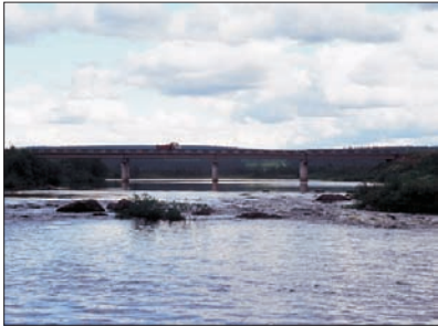
Fig. 5. View of the bridge upstream of sampling site K4, at Kitsa River. Photo: Tero Väisänen.
