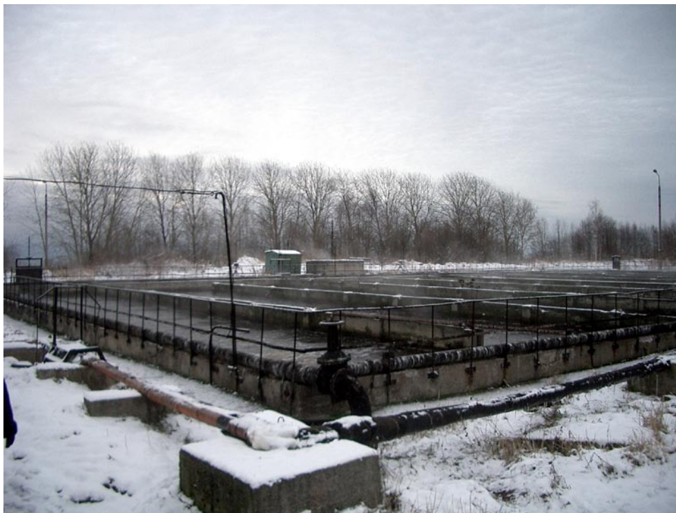
Figure 4.6. A view from the wastewater treatment plant of Petrozavodsk.
