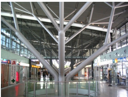
Figure 1. Image of the interior of Stuttgart Airport. Image shown is between Terminal 1 and 3 and was taken on 2005-06-02 by James Bowes and seen at http://en.wikipedia.org/wiki/File:Stuttgart_Airport_Interior_2005-06-02.jpg#filelinks .
