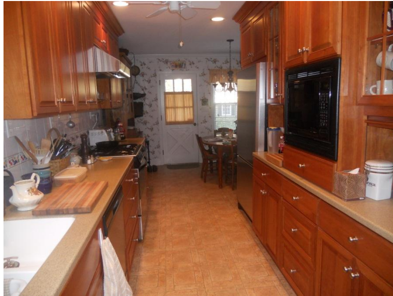
Figure 7. House #1 Kitchen Expansion. The rear exterior wall was removed in order to extend the kitchen out and include a breakfast area overlooking the back porch and yard. The original kitchen ended where the refrigerator now begins (Source: Author).
