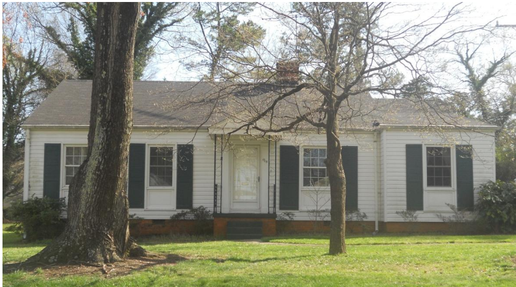
Figure 5. House #3 Exterior View. The Minimal Traditional style of the post-war era is characterized by low-pitched roofs, eaves with little to no overhang, minimal decoration and ornamentation, and is generally one-story (Source: Author).
