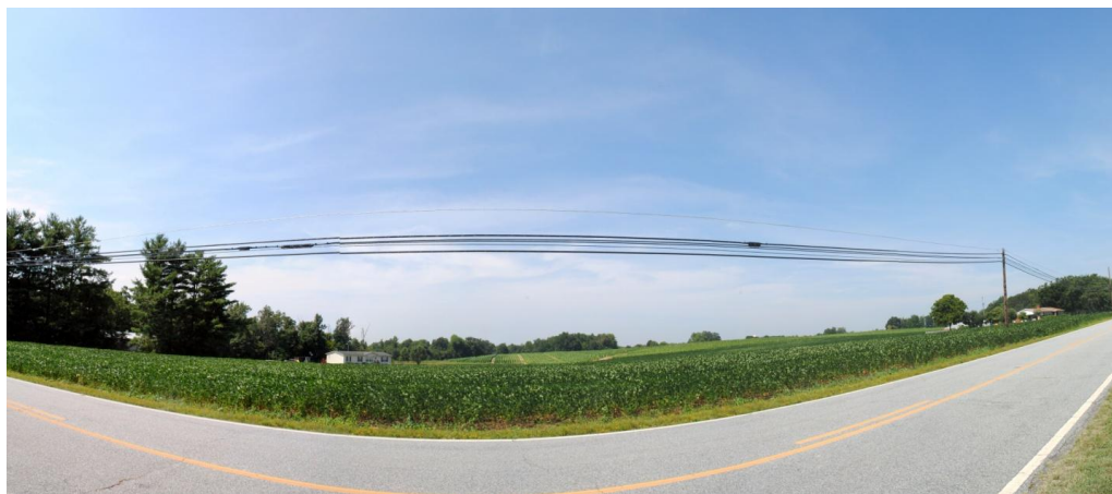
Figure 27. Suitable Site 3 Panorama. A panoramic view of Suitable Site 3 from the nearest roadway directed towards the center of the suitable site.
