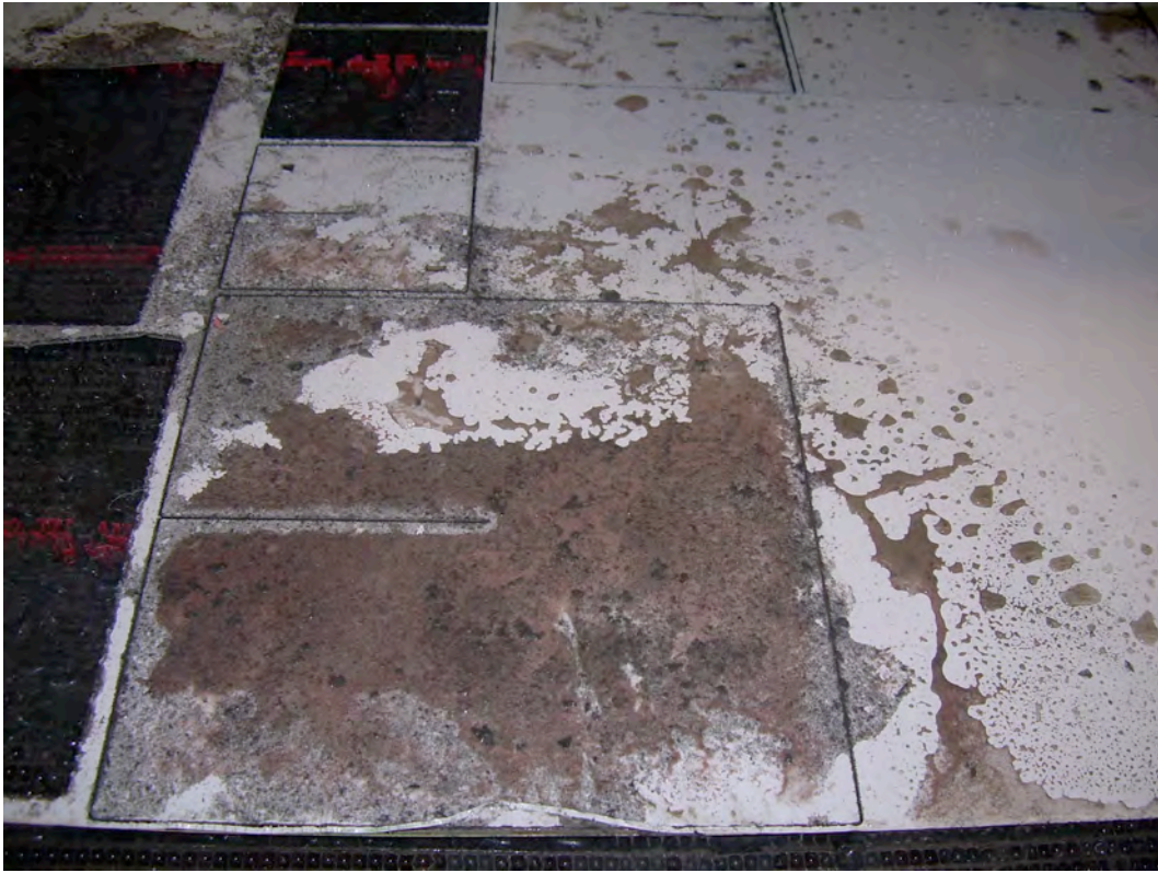
Figure 114: Water-jet cutting holes for spot welds.
