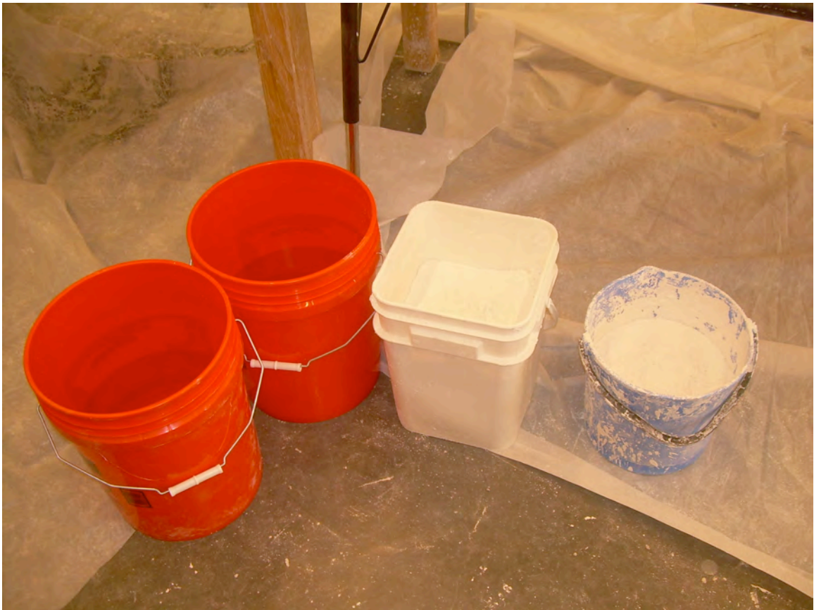
Figure 87: Dry mix prepared for mixing plaster.
