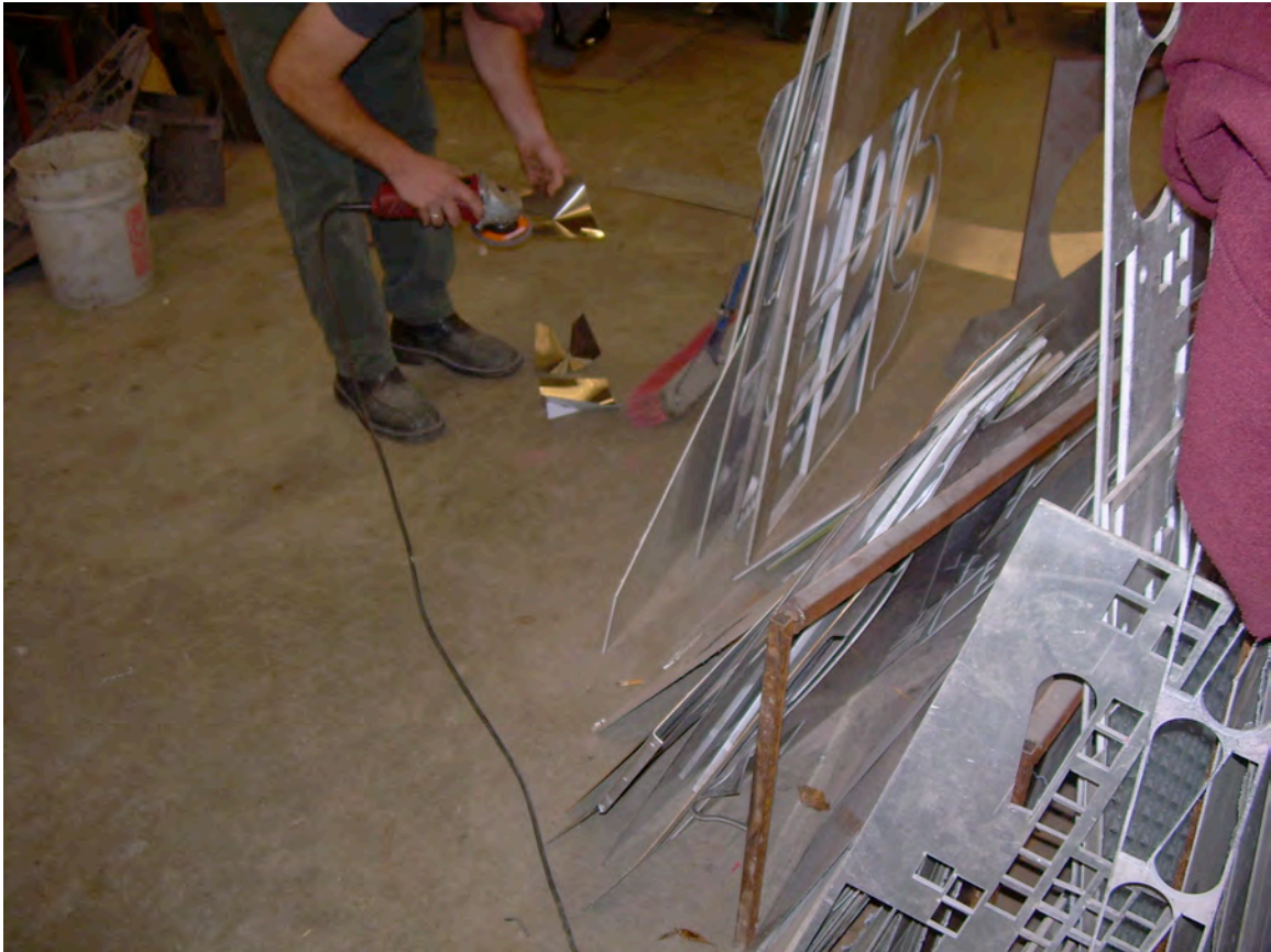
Figure 67: Sharp edges of sheet metal filed with an angle grinder.
