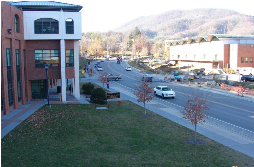
Figure 37. Third Daytime Area of Interest, Rivers Street Parking Deck, Looking Northwest.
