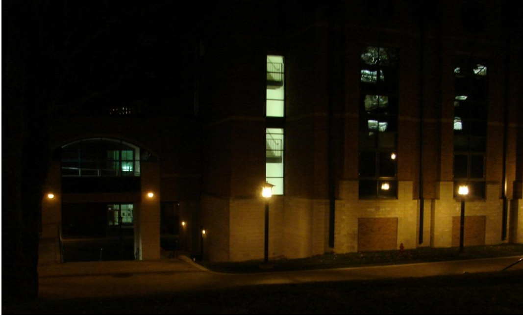
Figure 40. Second Nighttime Area of Interest, Front Entrance of Smith-Wright Hall, Looking West Towards Rankin Science North.
