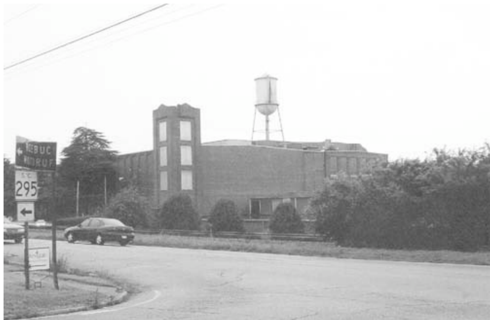
Figure 40. Arcadia Mill No. 2 Before Rehabilitation
