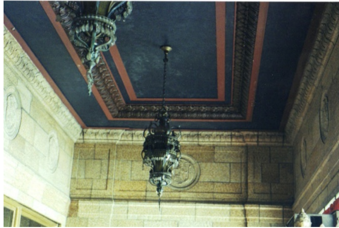
Figure 34. Tennessee Theatre, main foyer ceiling prior to rehabilitation
