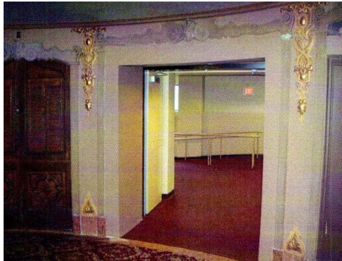
Figure 13. Stanley Theatre, orchestra level, lobby area wall removed to gain access to new addition off south exterior elevation; affected form, proportion, rhythm, and scale
