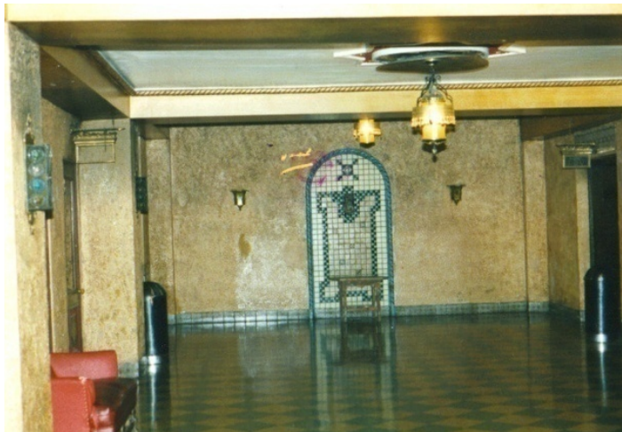
Figure 14. Tennessee Theatre, basement lobby area prior to rehabilitation
