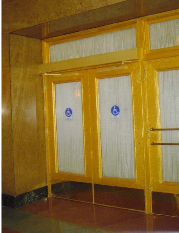
Figure 8. The Tennessee Theatre installed automatic doors to comply with ADA standards
