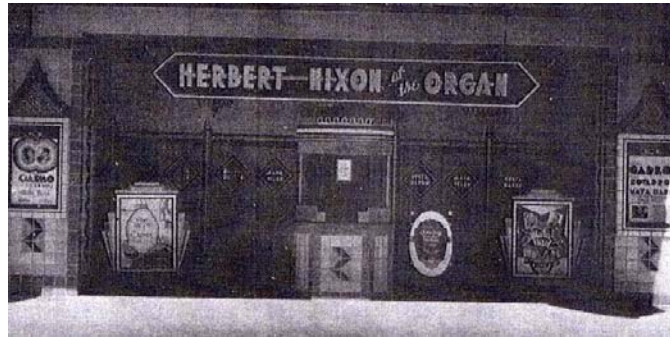
Figure 20. Fox Tucson Theatre, main entrance, historic photograph
