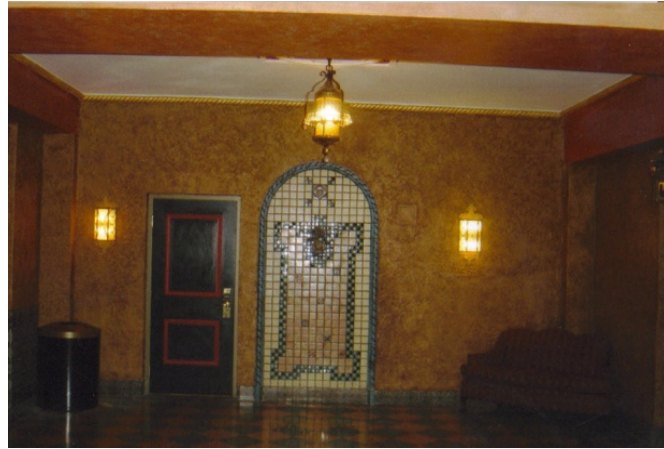
Figure 15. Tennessee Theatre, a door was added on the east wall of the basement lobby to access the corridor; affected rhythm
