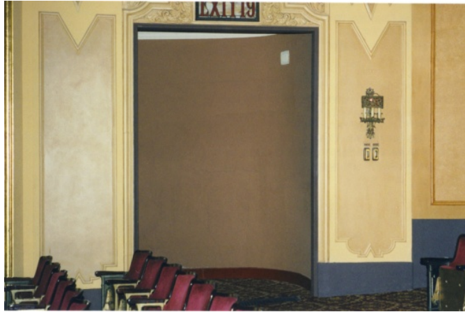
Figure 28. Stanley Theatre, auditorium side exit prior to rehabilitation
