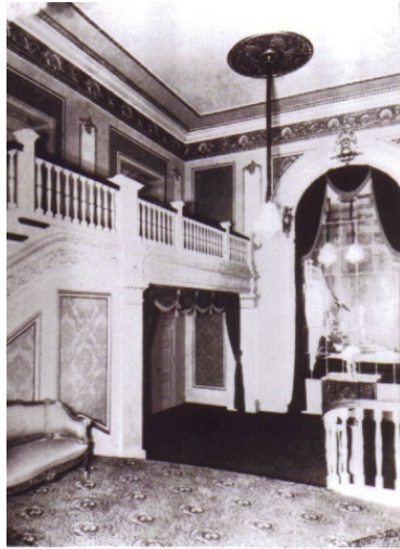
Figure 23. Missouri Theatre, grand foyer, historic photograph
