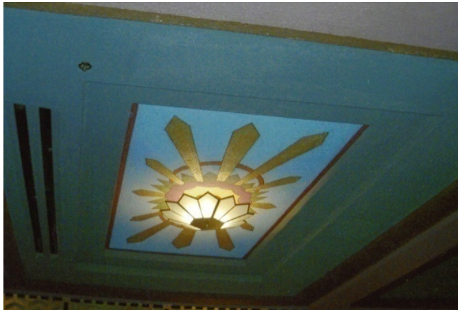
Figure 31. Fox Tucson Theatre, ceiling was repainted in the audience chamber
