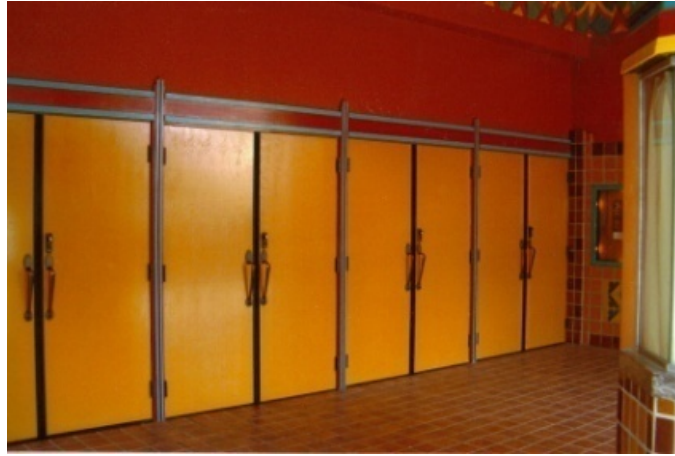
Figure 22. Fox Tucson Theatre, main entrance glass doors were replaced with solid doors prohibiting natural light from entering the lobby space
