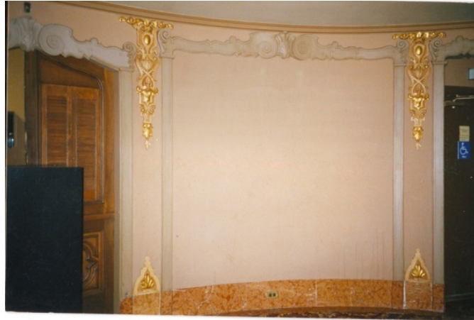
Figure 12. Stanley Theatre, orchestra level, lobby area prior to rehabilitation
