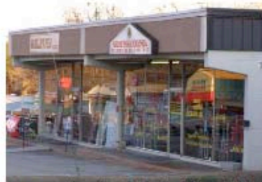
Large repetitive walls of glass should be avoided.
