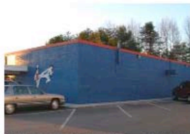
Painted concrete block and long unbroken walls with no detail are not appropriate for the commercial corridor.
