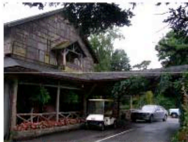
The natural materials used in this building help to define a positive sense of place and a consistent visual image that expresses local character.
