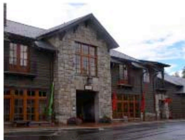
Stone, wood, and slate shingles provide a color scheme that reinforces the mountain village aesthetic.
