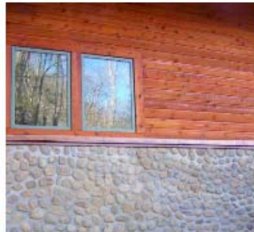
This is a good example of combining wood with stone, with the stone at the base level and the wood above.
