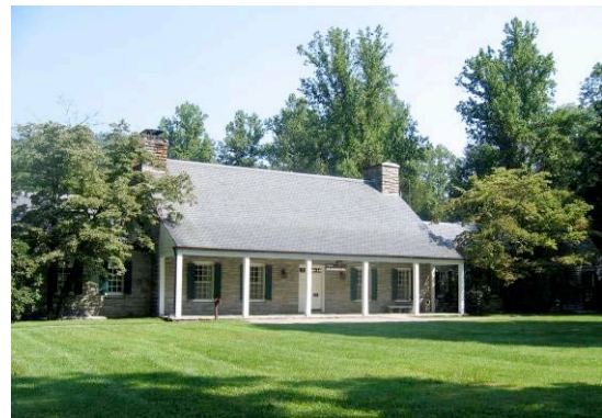
Figure 29. Sugarlands Administrative Office (1940). Photo taken by author.
