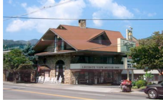
Figure 49. LeConte View Motor Inn. Photo taken by author.
