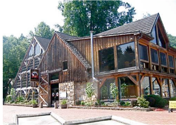
Figure 20. New Development: Calhoun's Village. Photo taken by author.
