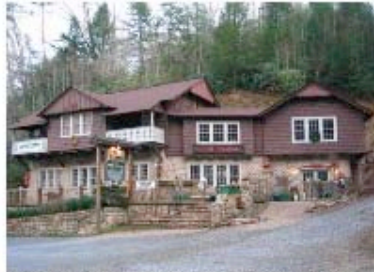
The building cascades down to the front of the site and the building massing is broken up into smaller units.
