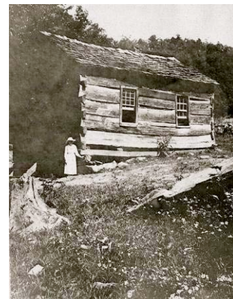
Figure 9. Pi Phi's neighbor, up Baskin's Creek.
