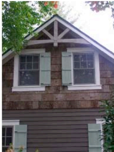
This building creatively uses two variations of wood to break up the vertical masses.
