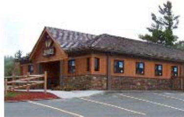
This building takes advantage of different shades of wood and stone in order to create a rustic appearance.
