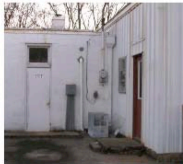
Unattractive utility areas like this should be screened so that they cannot be seen from the street.
