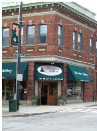
Well-designed awnings provide a way to present signage and identify a business without interfering with the public way.
