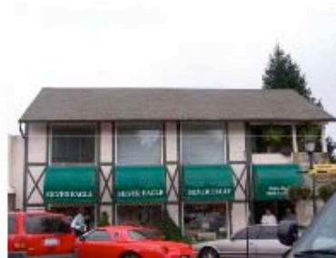
The lack of variation in the massing of this building detracts from its appearance.
