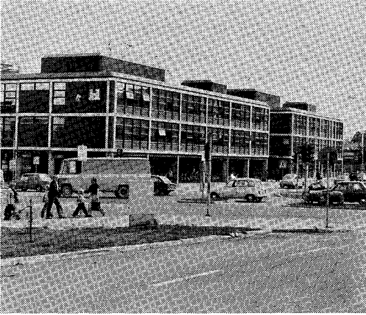
Fig. 8. View from the test catchment Kajaani centre.
