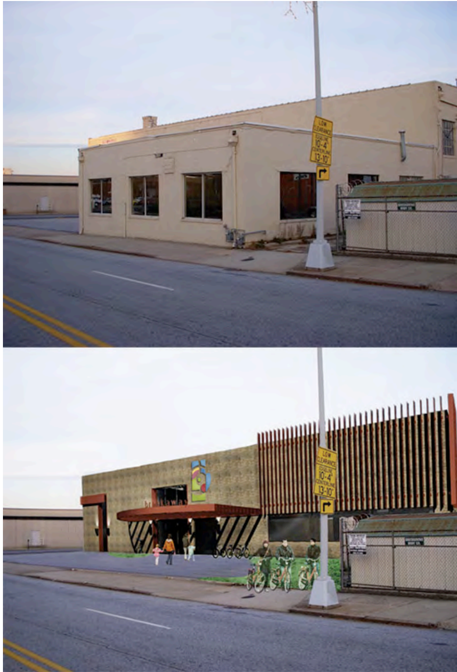
Figure 29. Before and after images of the west facade of 304 East Market Street, exposing the removal of the attached low building.
