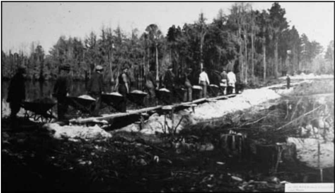
Image 7. Works Progress Administration at work at Greenfield Lake, 1932. New Hanover County Public Library
