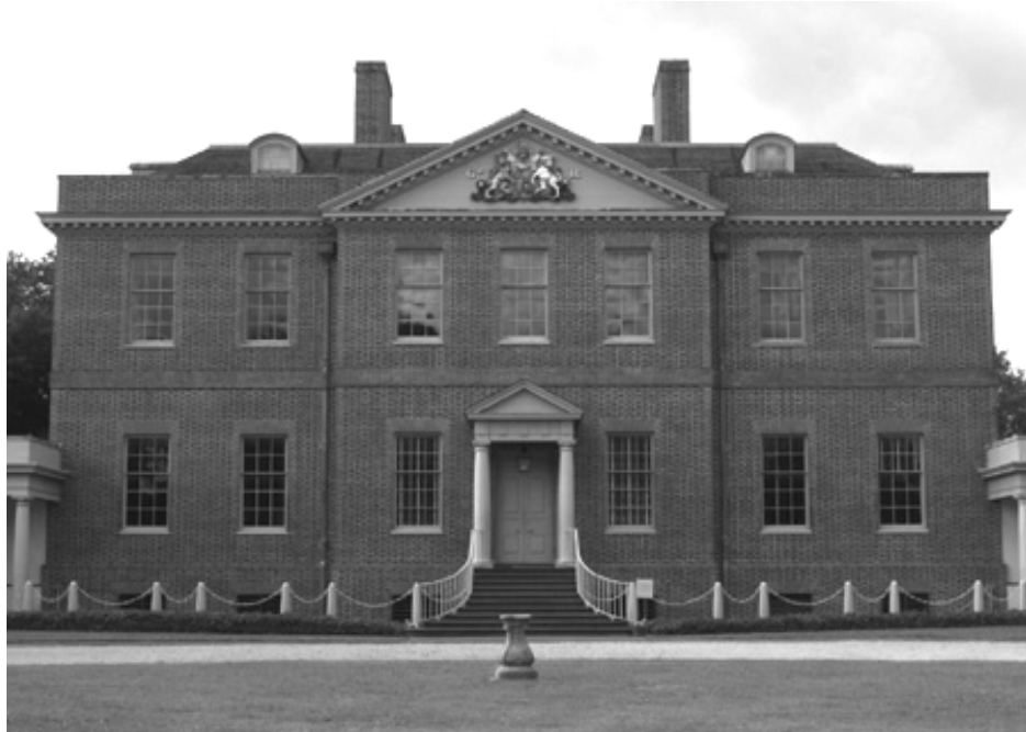
Figure 14. Front Elevation, Tryon Palace, New Bern, North Carolina, original design by John Hawks, reconstructed by William G. Perry, 1952-59. Photo by author.
