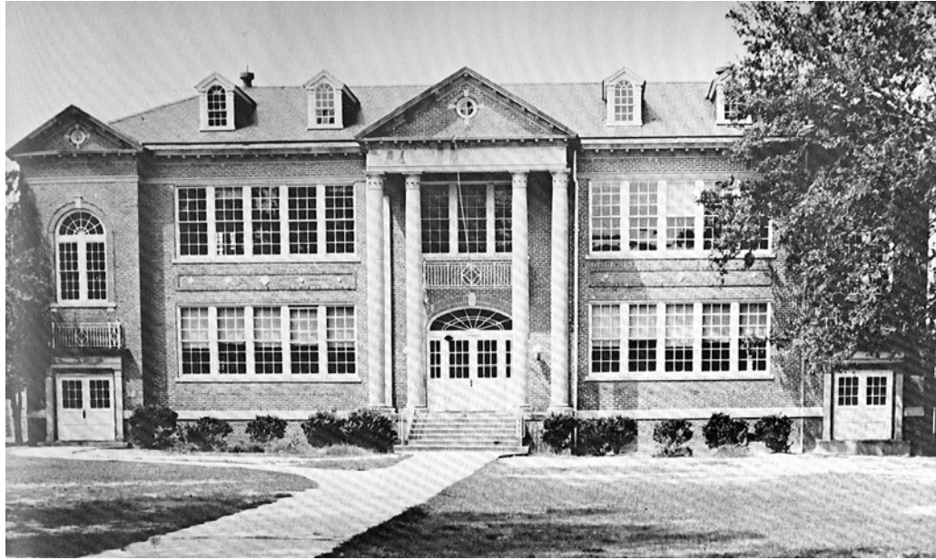
Figure 22. Moses Griffin Building, 1930, designed by Leslie N. Boney, Sr. of Wilmington. From Green, A New Bern Album , p. 291.
