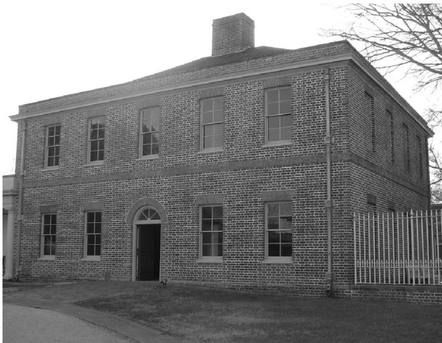
Figure 11. Restored West Wing, 2005, New Bern North Carolina, original architect John Hawks, 1767-1770, restoration architect William Graves Perry. Photo by author.
