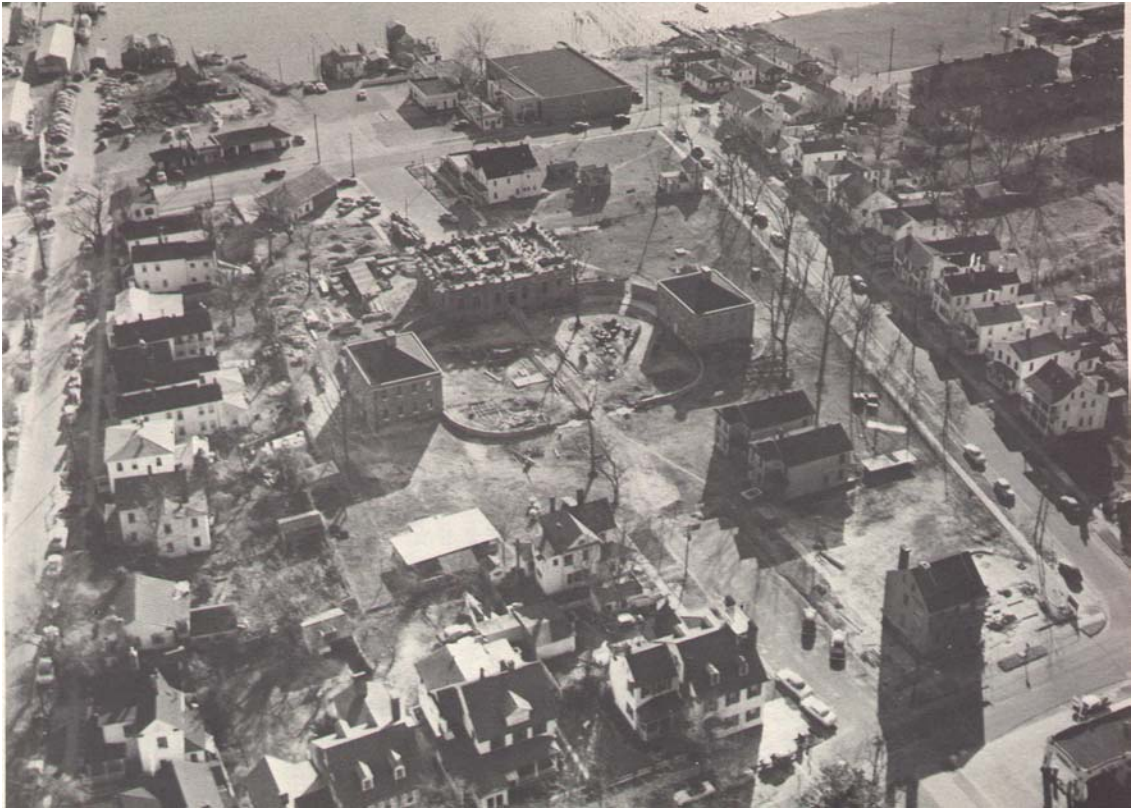
Figure 16. Aerial view, Palace restoration, January 3, 1956. From Robinson, Three Decades of Devotion , p. 86.
