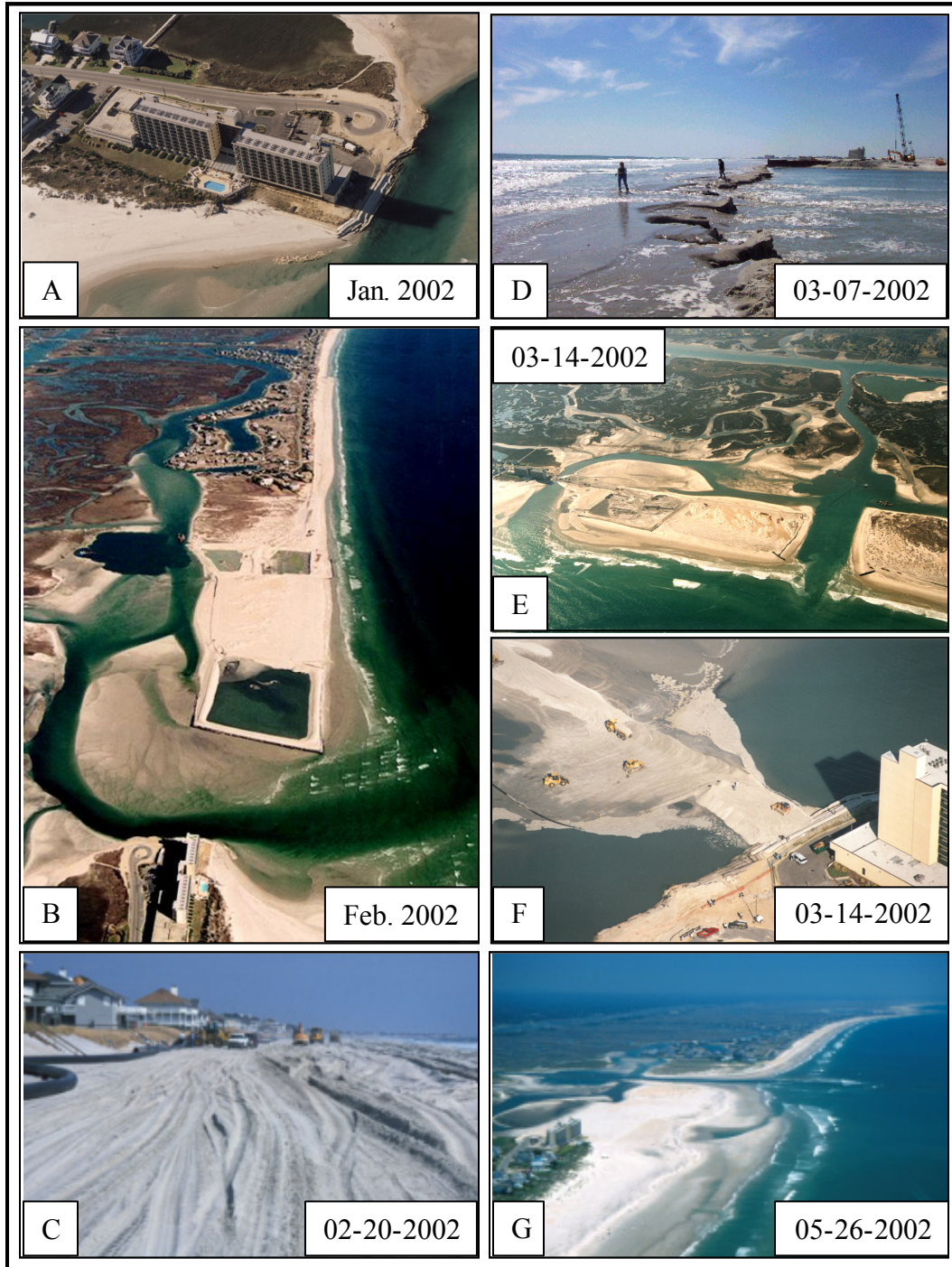
Figure 2. Photographs illustrating (a) Shell Island Resort, (b) construction phase, (c) beach nourishment of Figure Eight Island, (d) inlet opening, (e and f) old inlet closure, (g) original inlet closed and ebb shoal collapse, associated with the relocation of Mason Inlet. Photographs courtesy of ATM and Dr. W. Cleary.
